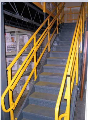
Code-compliant stairs and landings
